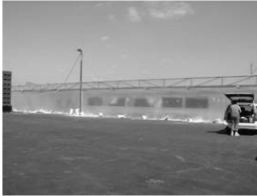
Fig. 3. General view of the drier consisting of a green house.
